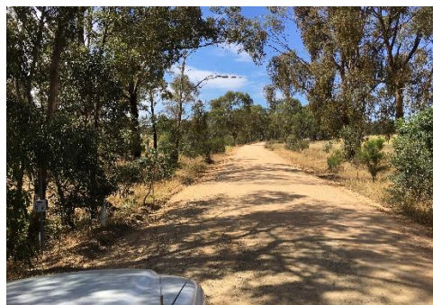
(a) S4 trial road section before stabilization
