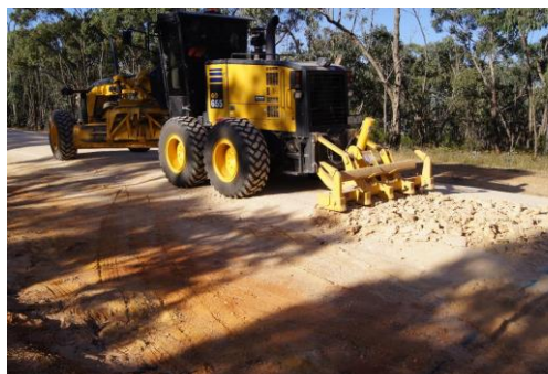
(b) Stage 1: Ripping of trial section with grader
