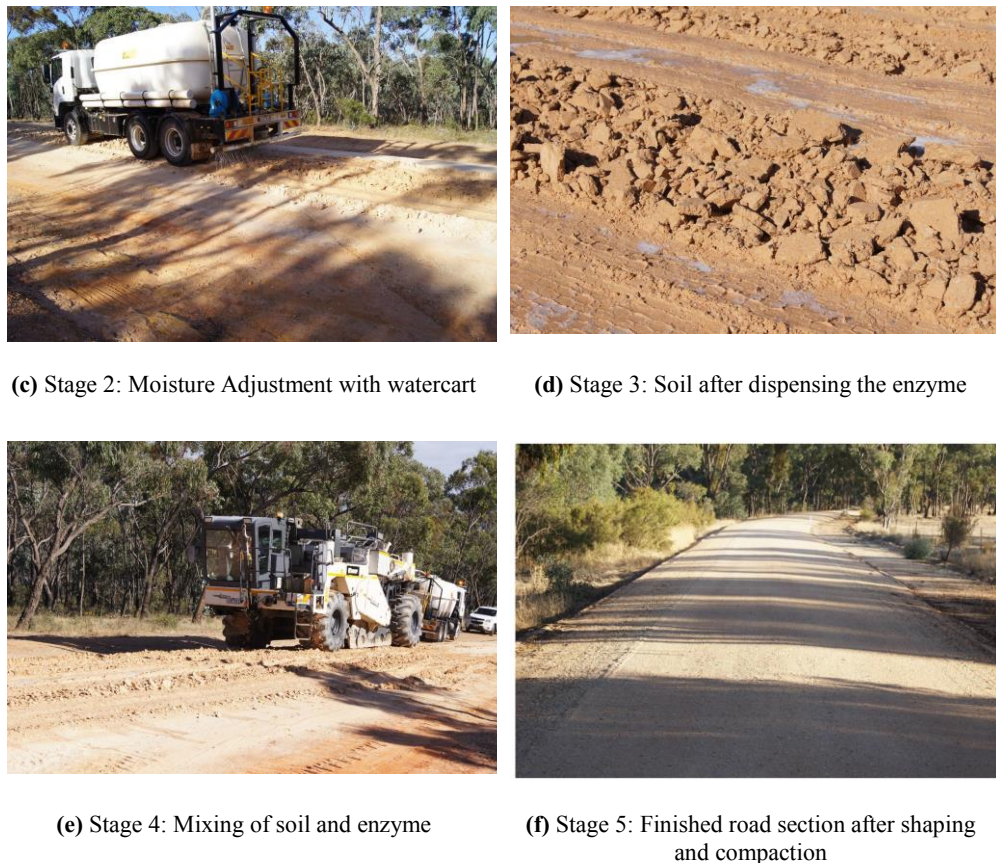
Fig. 3. Construction stages of trial road construction
