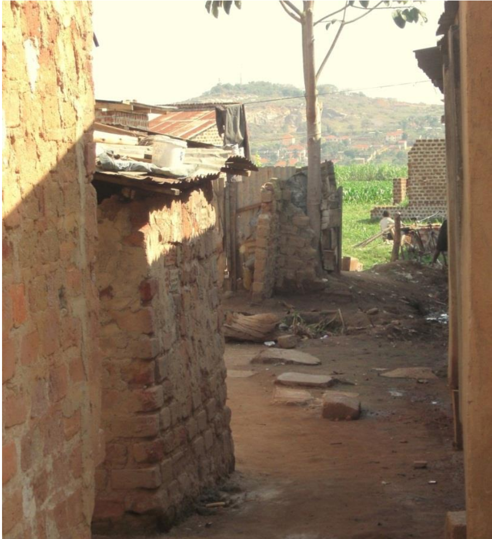
Plate 1. Typical one-roomed dwellings in Kiweranga, made with locally-made mud bricks, and built on encroached wetlands. Photo taken by author.
