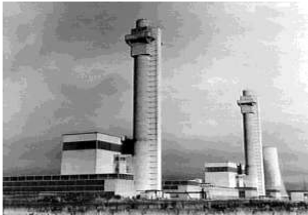
a) Air cooled chimneys of the Windscale Plutonium Pile
