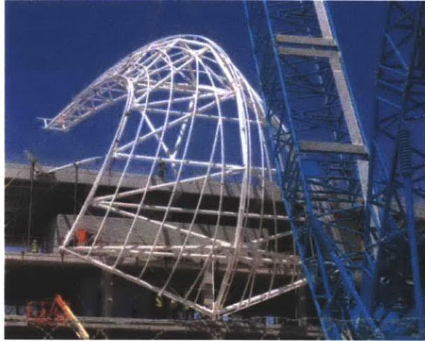
Figure 51: Roof Girder Installation (Nelson Mandela Multi-Purpose Stadium 2010)
