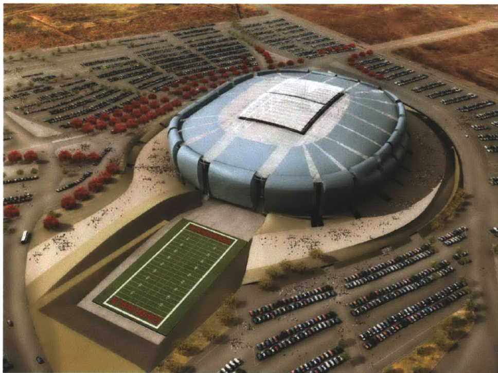
Figure 43: Arizona Cardinals Stadium (World Stadiums 2012)
