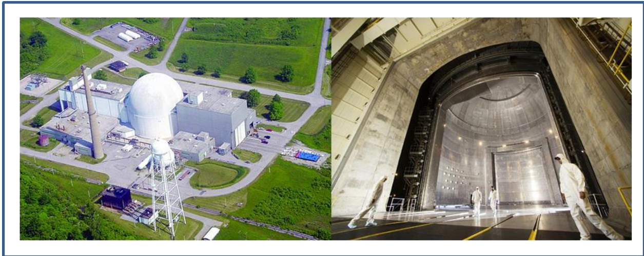
Figure-7- Plum Brook Station Test facility and a view of the TVAC Chamber
