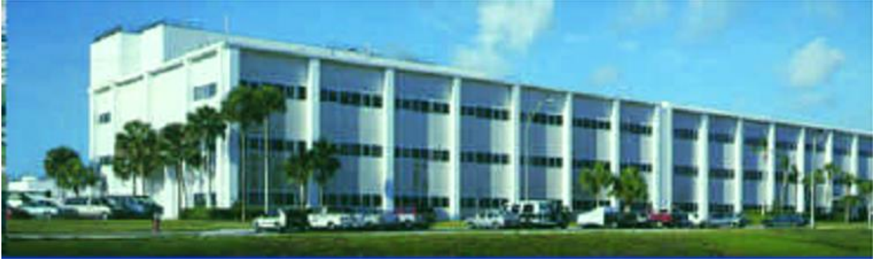
Figure 1 - Neil Armstrong Operations & Checkout Building (O&C) at KSC Industrial Area
