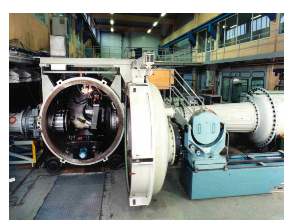
H2K wind tunnel, with test section open
