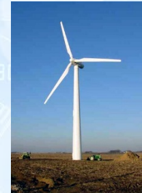
Wind Turbine Doubly Fed Machine
