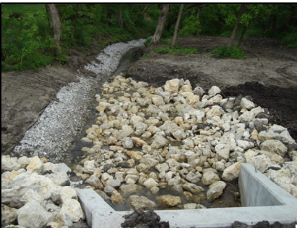
Photo C - Outlet of Storm Water Detention Basin
