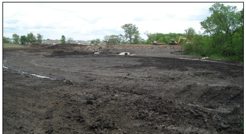
Photo D - Storm Water Detention Basin & Vegetative Buffer
