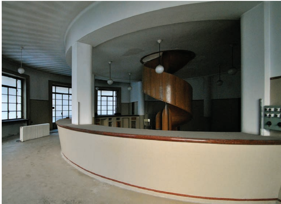
Fig. 14. Interior of the reception office of the former Sanatorium Village in Sondalo before restoration, 2012
