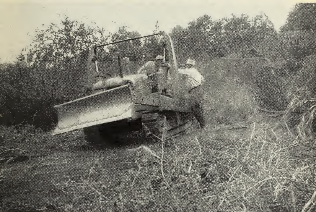
Fig. 4—Same field as in figure 3. Above, close-up showing the brush knocked down and left in place. The result is an even distribution of the ash after the dried brush is burned. Below, equipment used for knocking down brush. The blade of the bulldozer has been raised in order to turn around. Note the soil has not been disturbed. (Photographed May 15, 1946)
