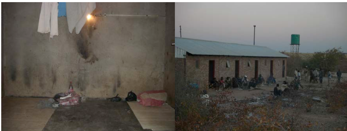
Left: Inside a New Houses room; Right: the Hostel
