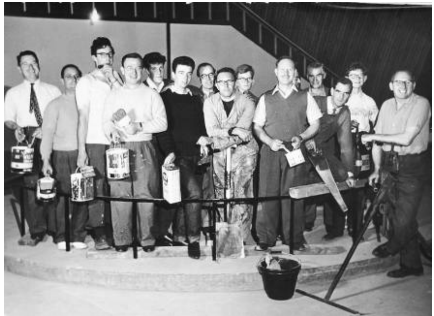
Top left: The shell roof structure had to be made in wood before being cast in concrete and the temporary timber was self-supported on a forest of scaffolding. Photograph in Chatburn, 1990.
