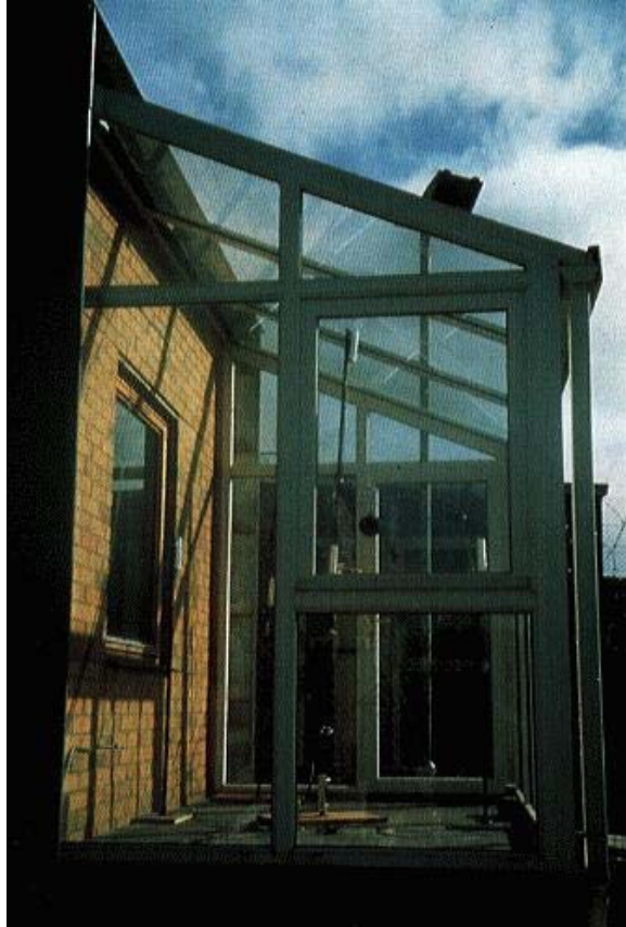
Figure 9: Conservatory installed on south wall of test cell
