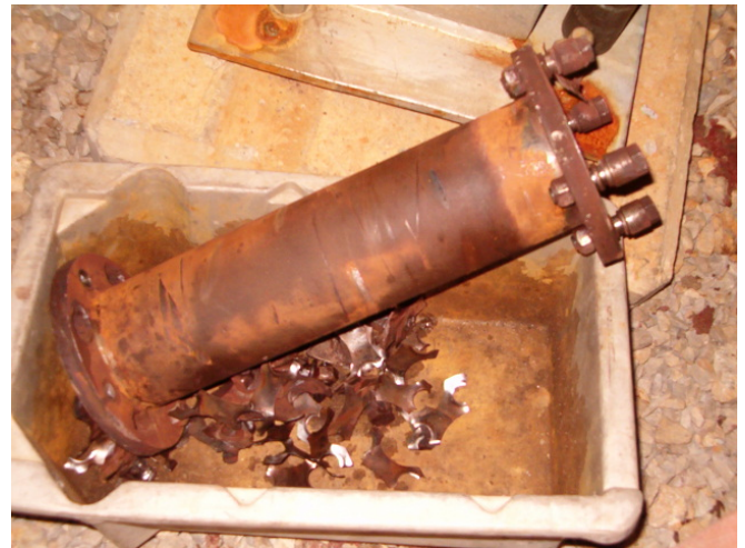
Figure 53. Coupling spool piece which ejected from the machine.
