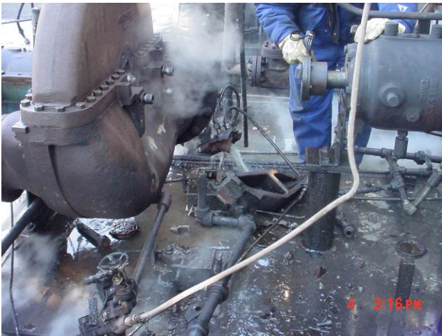
Figure 13. Damaged Turbine
