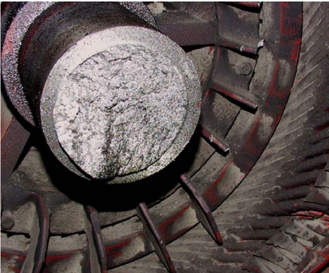
Figure 82. Close up of fractured motor shaft
