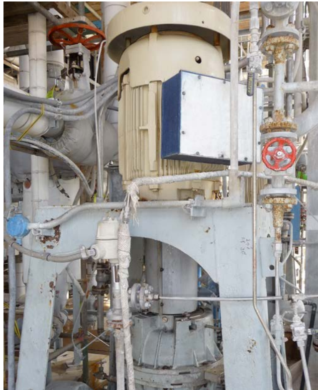
Figure 54. Vertical compressor with 3590 RPM motor.
