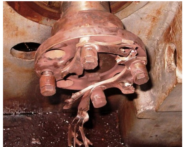
Figure 52. Turbine hub disc pack sudden fracture.
