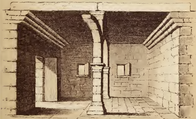
INTERIOR SHOWING STONE ROOF.
