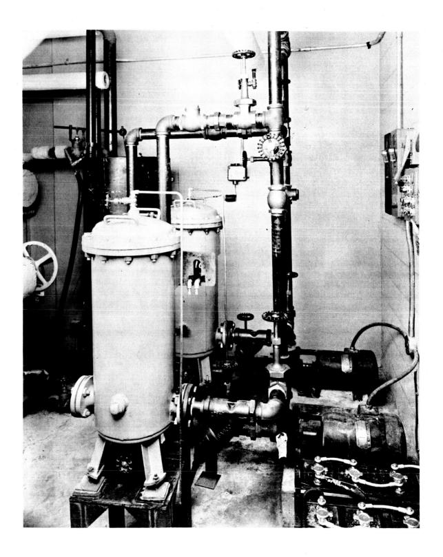
FIGURE 10 FILTERS IN WATER-COOLING SYSTEM
