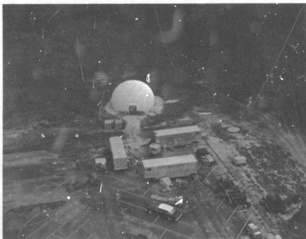
Fig. 2. Typical mobile station
