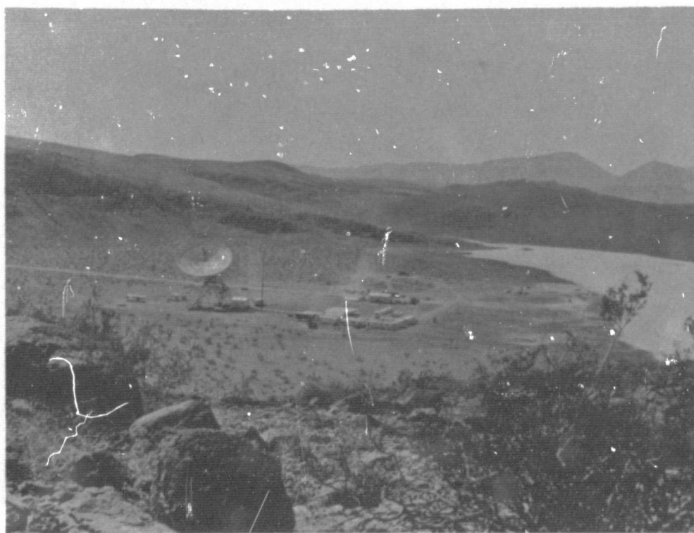
Fig. 1. Typical Deep Space Station (Goldstone receiver site)
