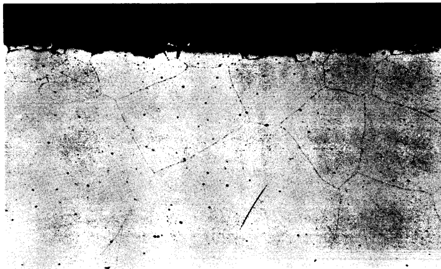
Figure 59. Appearance of the Crack Found in the Tube Wall of the Superheater After 262 Hours of Operation.
