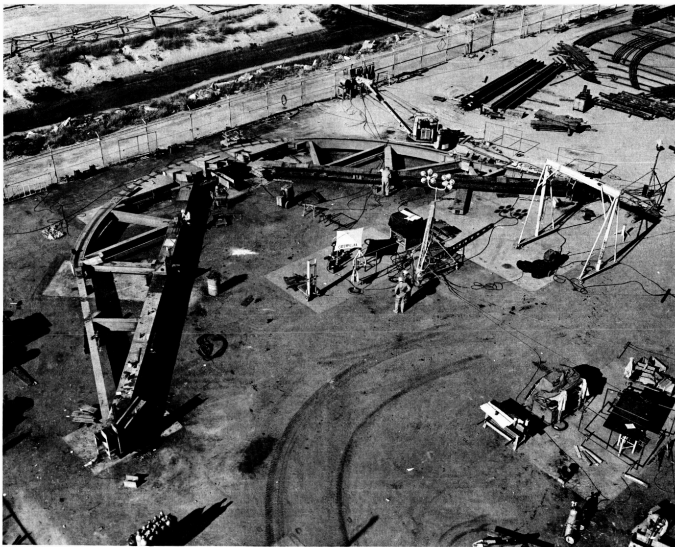
Fig. 11. Elevation wheel truss fabrication
