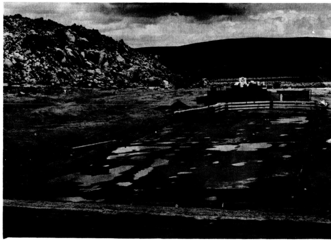
Fig. 7. Floor slab of the bulk stores building
