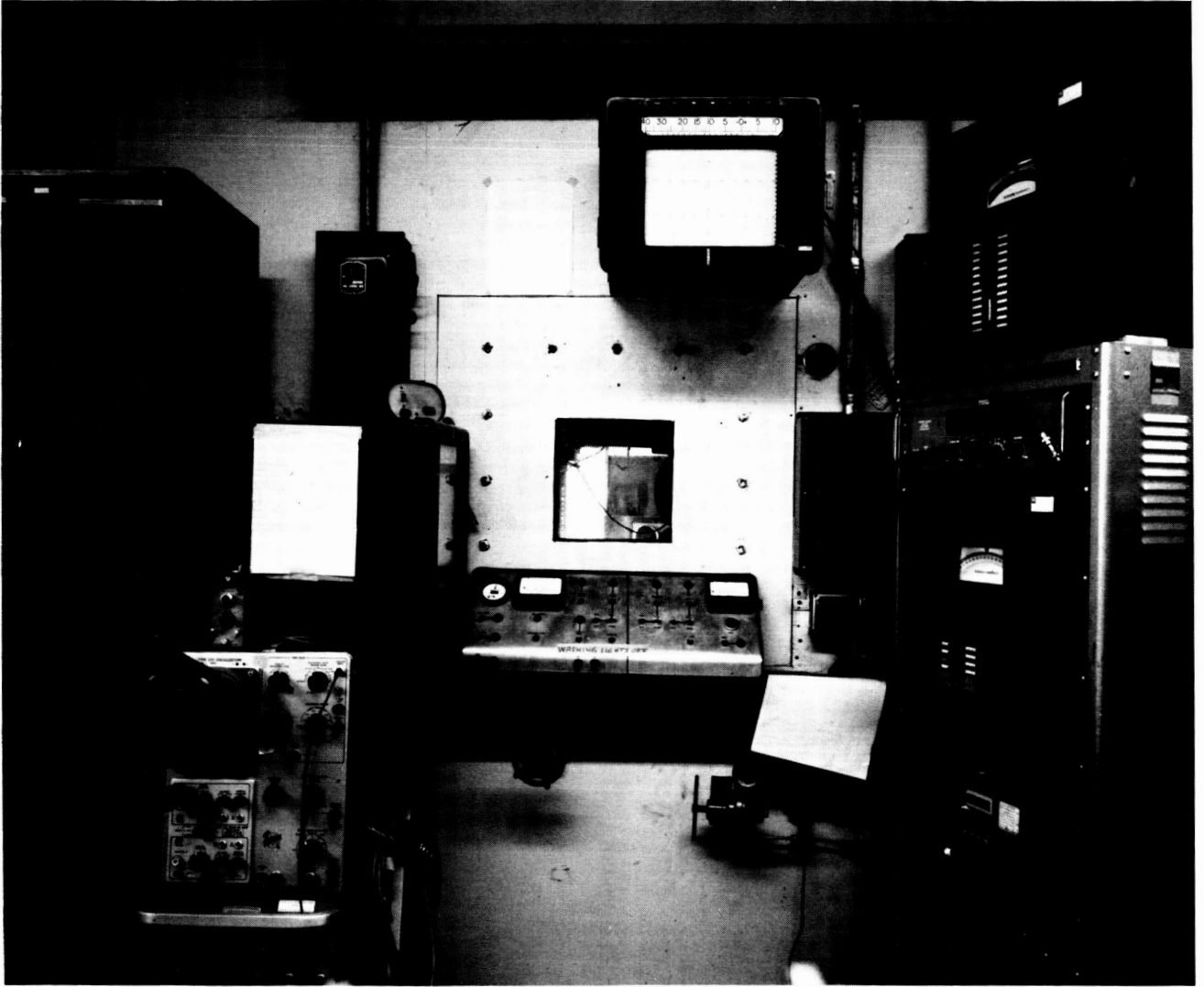
Fig. 3-32 - Engine Control Room
