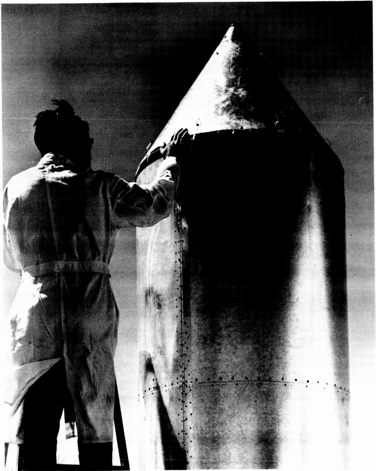
FIGURE 82 - ONE-FOURTH SCALE MODEL USED FOR PATTERN STUDY
