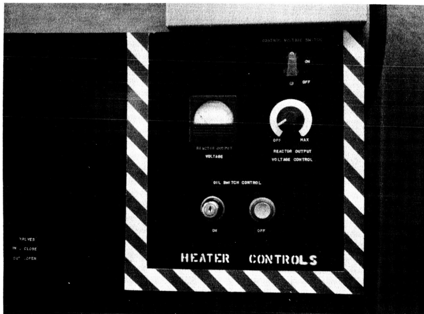
Figure 34 - Power Supply Control Panel
