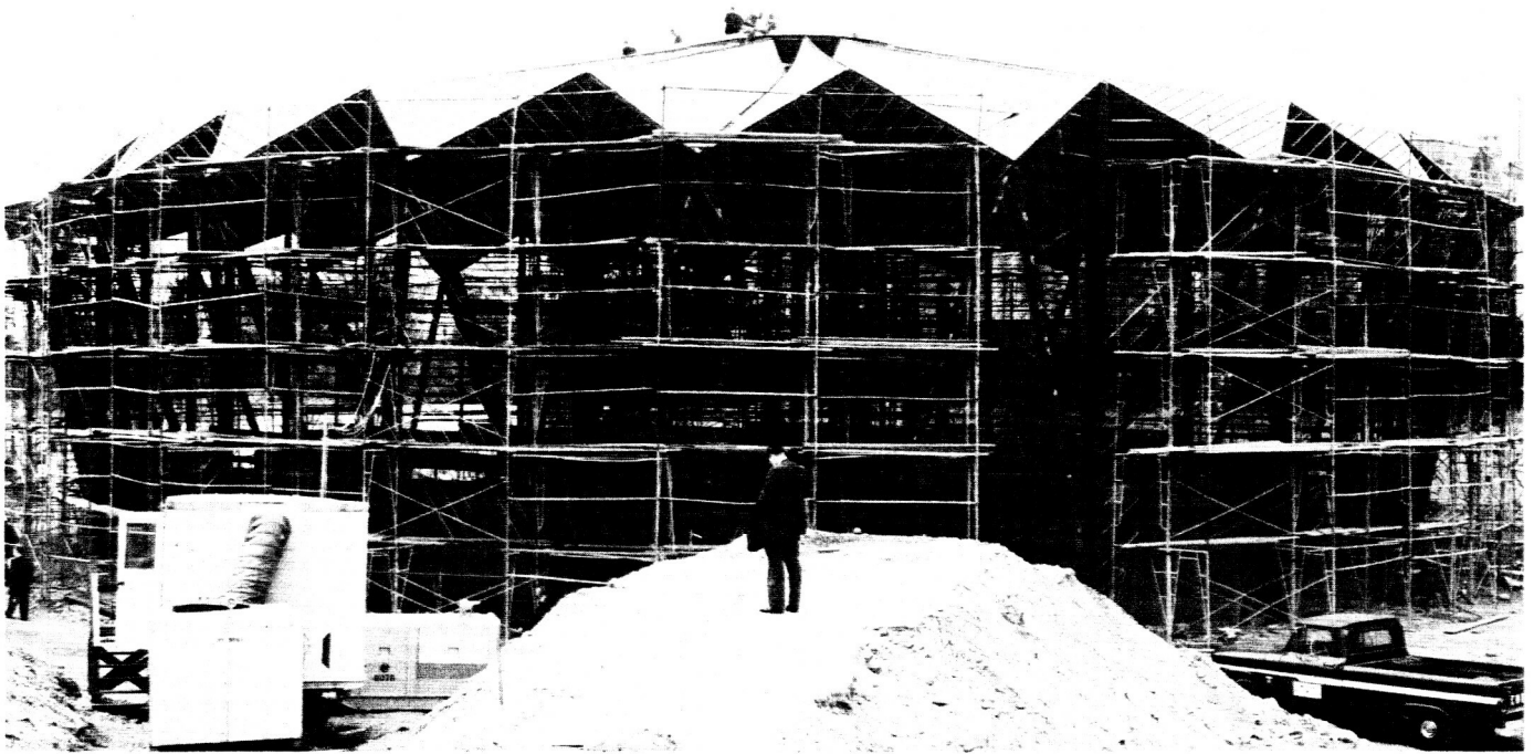
Fig. 11. JPL instrumentation trailer, with portable power supply and air conditioning units, at construction site
