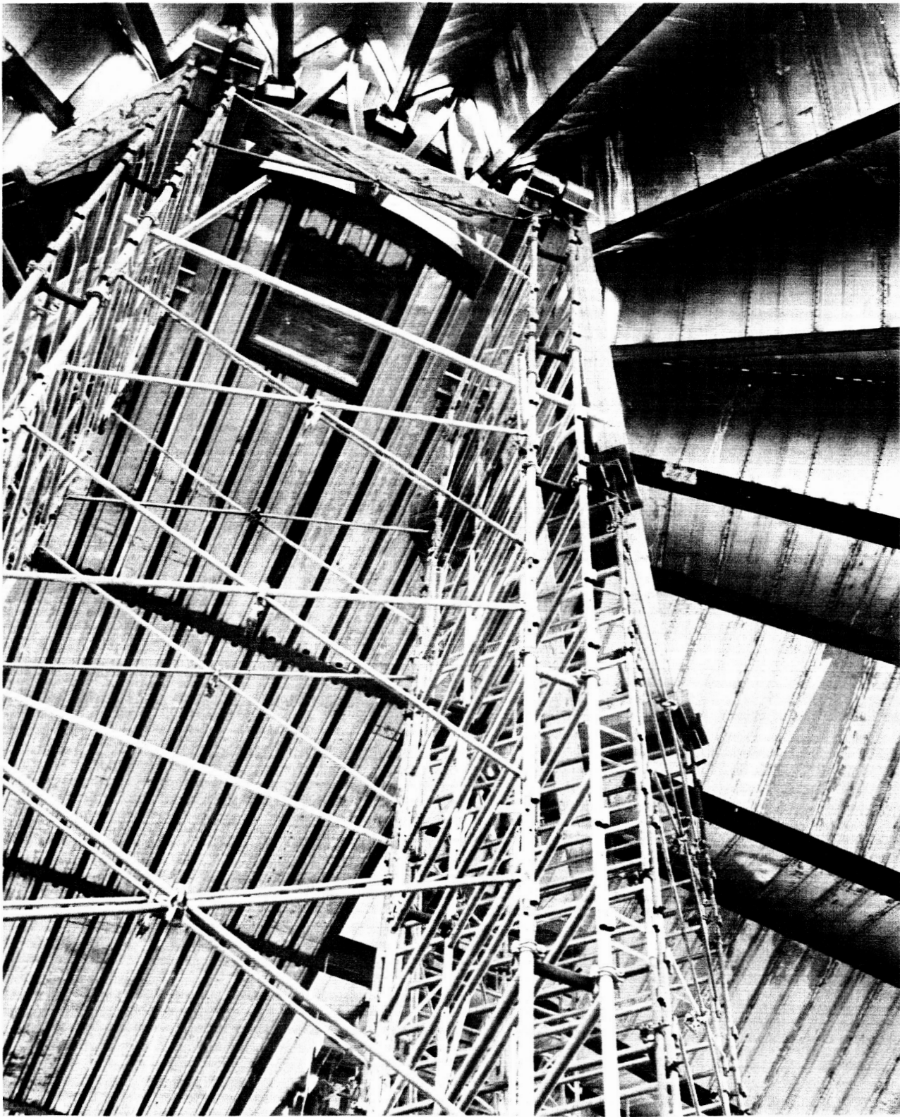
Fig. 3. Facility equipment platform supported by jack array
