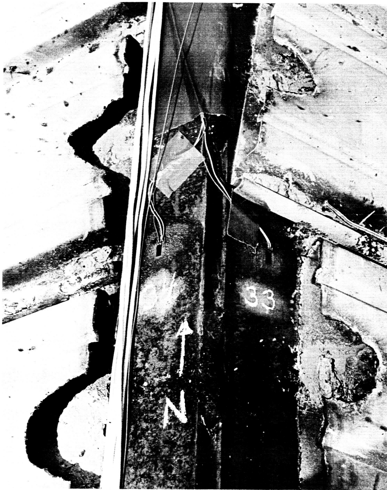
Fig. 7. Strain gauge installation on roof fold-line member
