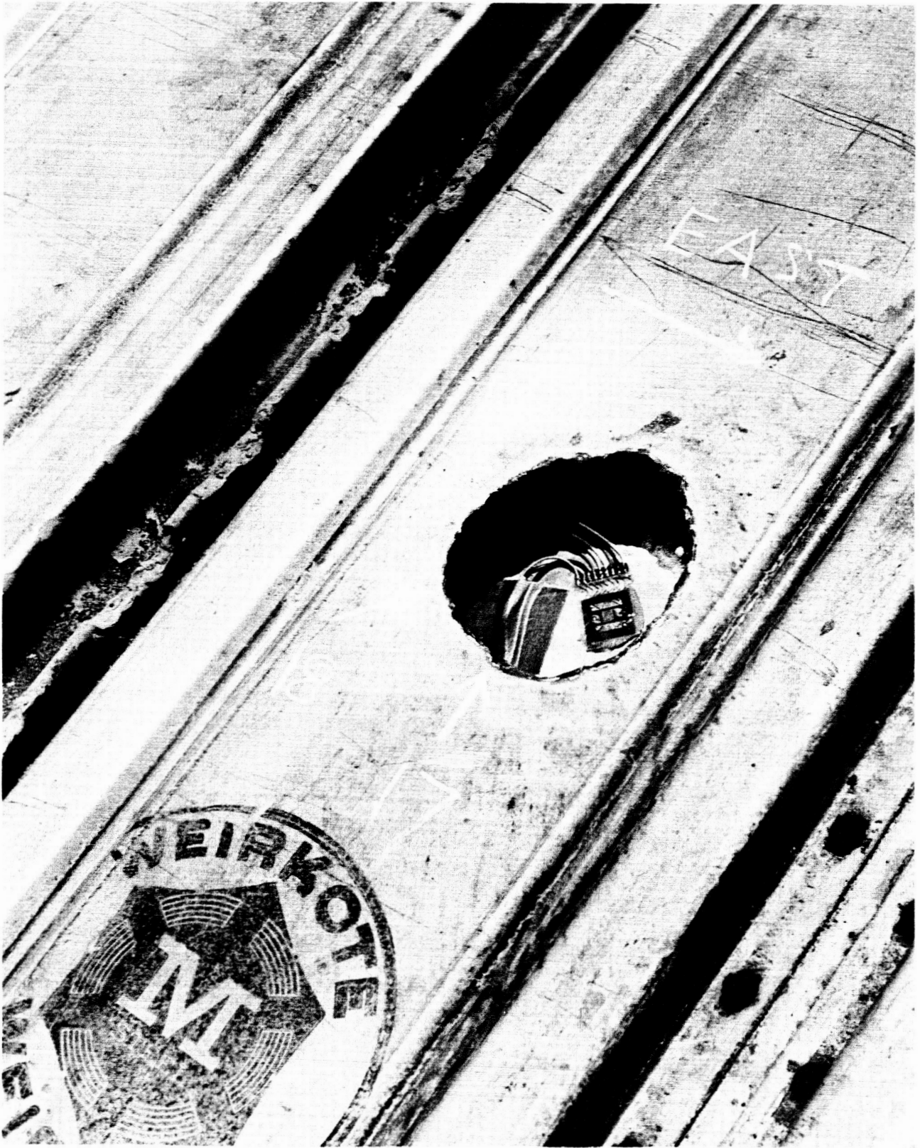
Fig. 9. Strain gauge installation on roof fold-line member along minor axis
