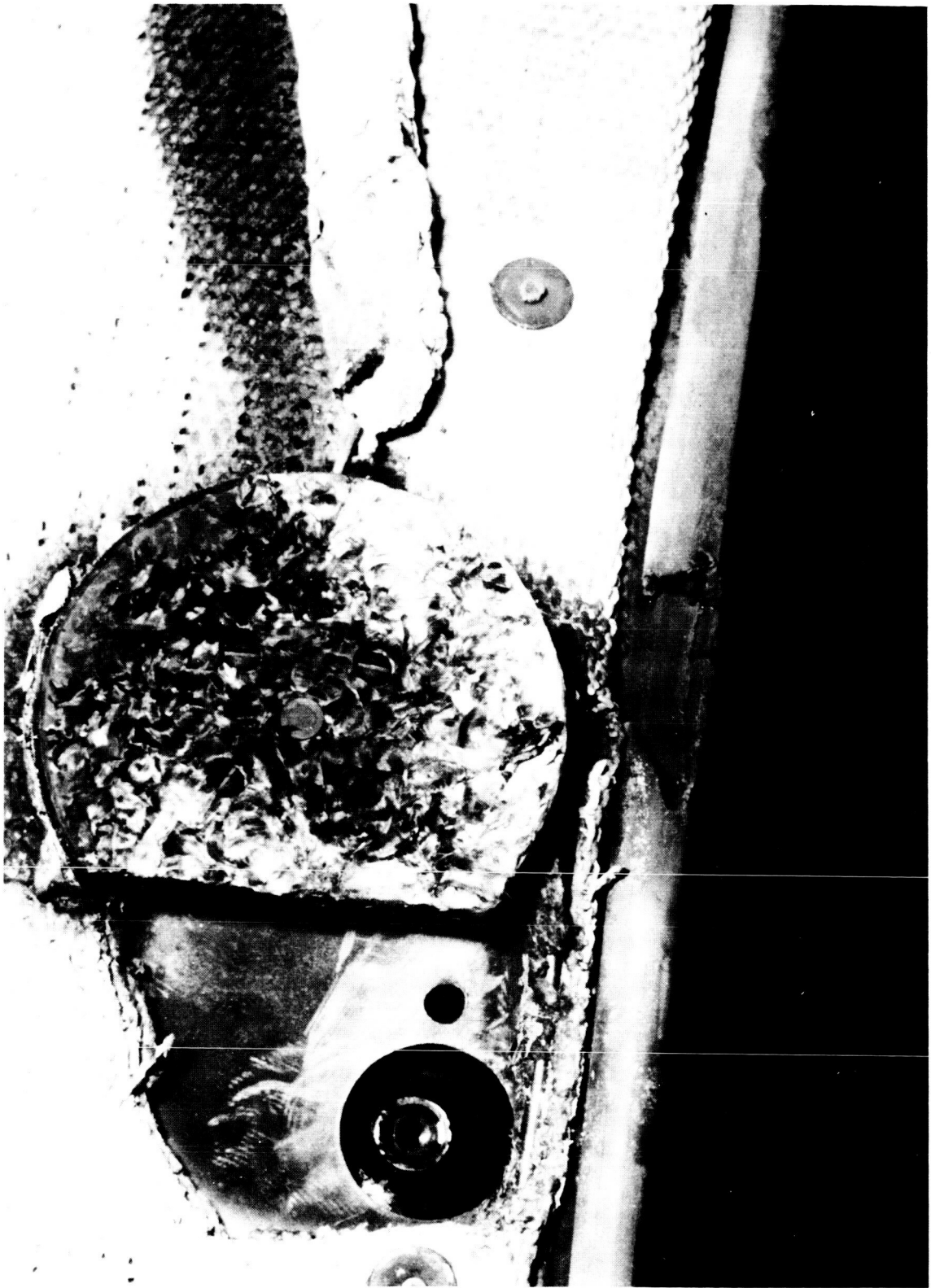
FIGURE 2-4 METAL EROSION, ASPIRATOR LIP OF ENGINE 3
