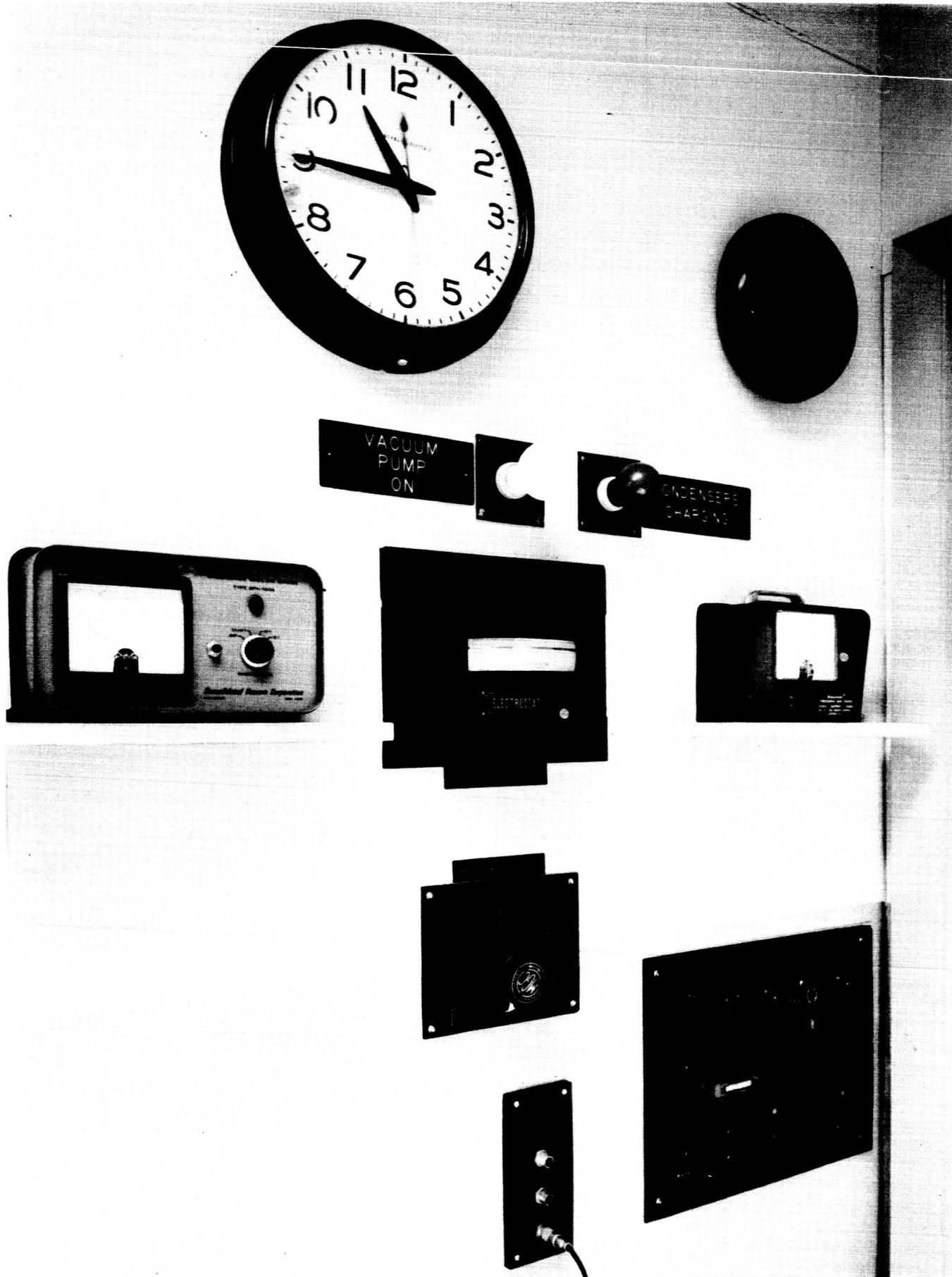
CONTROL PANEL FOR THE 155,000 JOULE CAPACITOR FORMING FACILITY FIGURE 40 65
