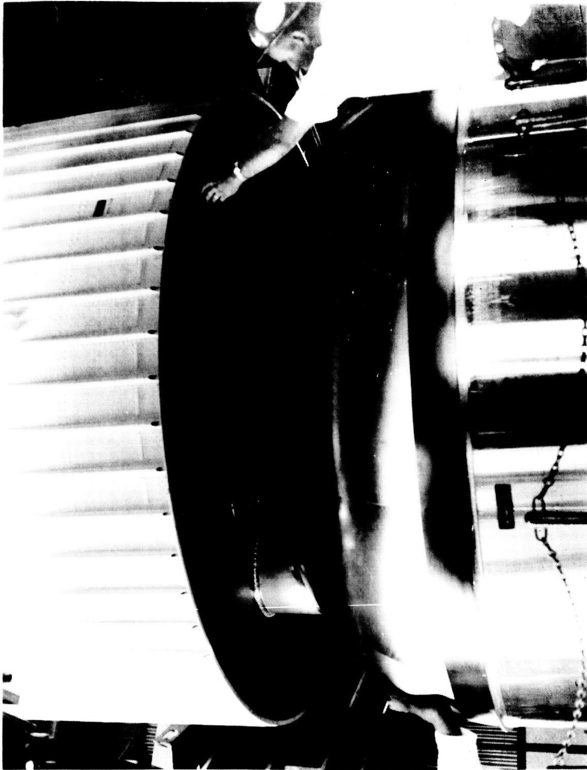
Figure 19.3-4. Interstage Adapter/Booster Mating
