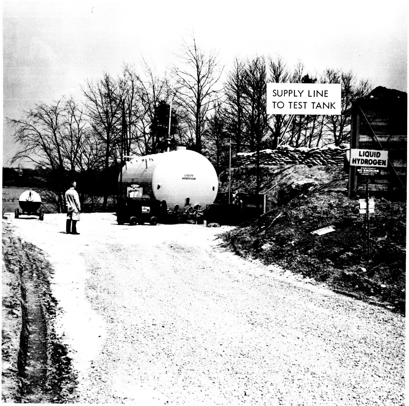
Figure 69. LH 2 Storage Tank at Rear of Test Bunker
