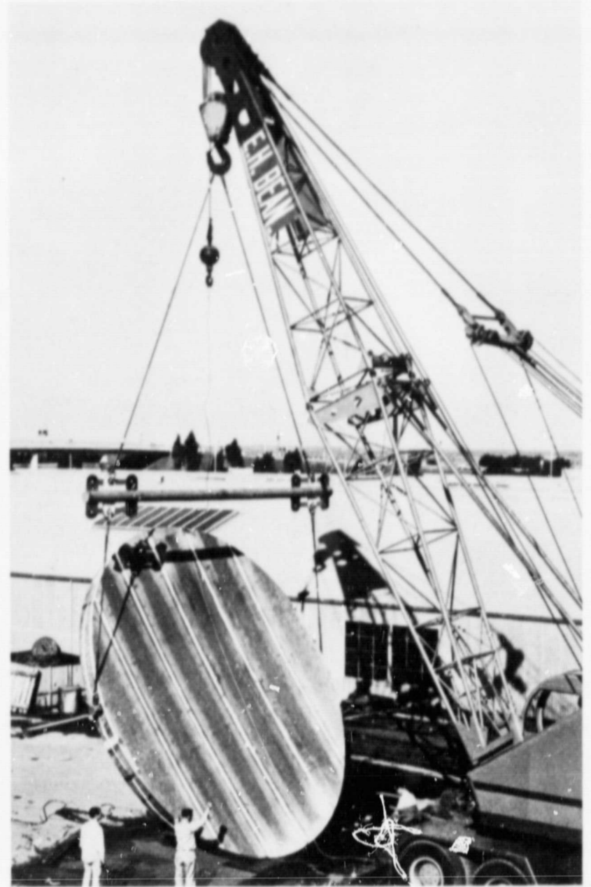
Fig. 15. Unloading mirror for creep-sagging weldment
