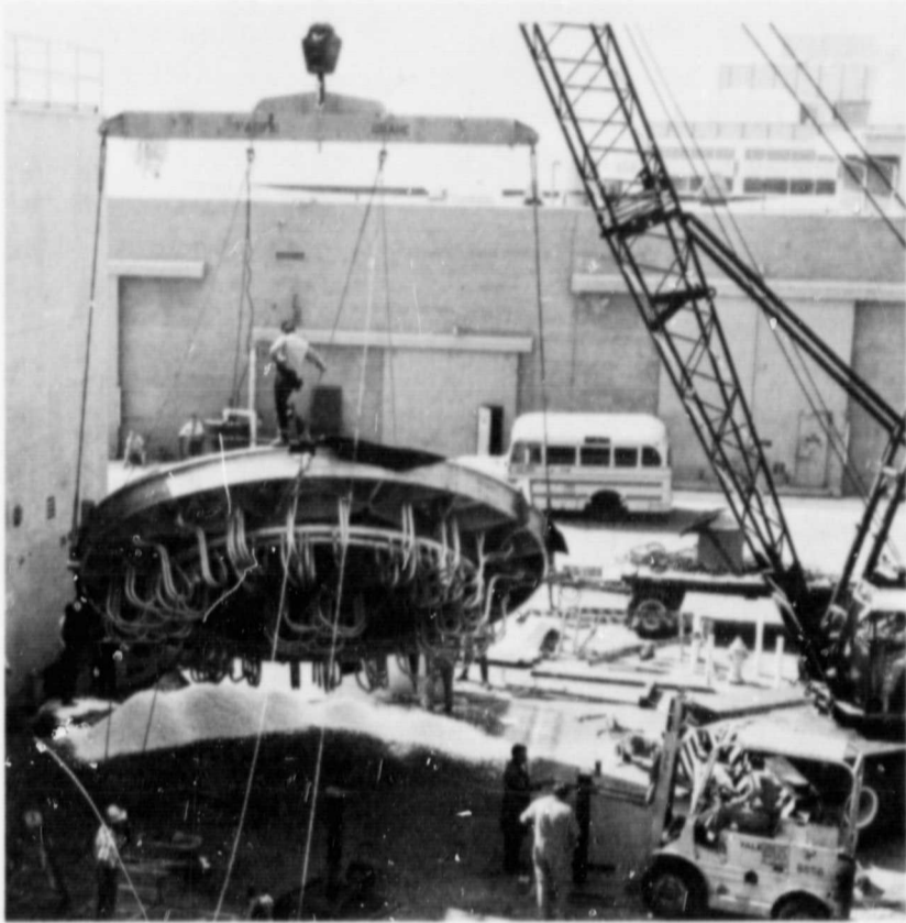
Fig. 28. Moving mirror onto handling cart
