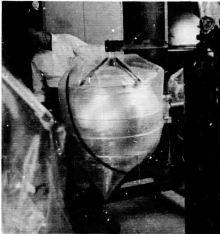
Fig. 4.2.1-35 VAPOR-COOLED SHIELD
