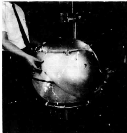
Fig. 4.2.1-26 SHIELD UNDER ALL BUMPERS
