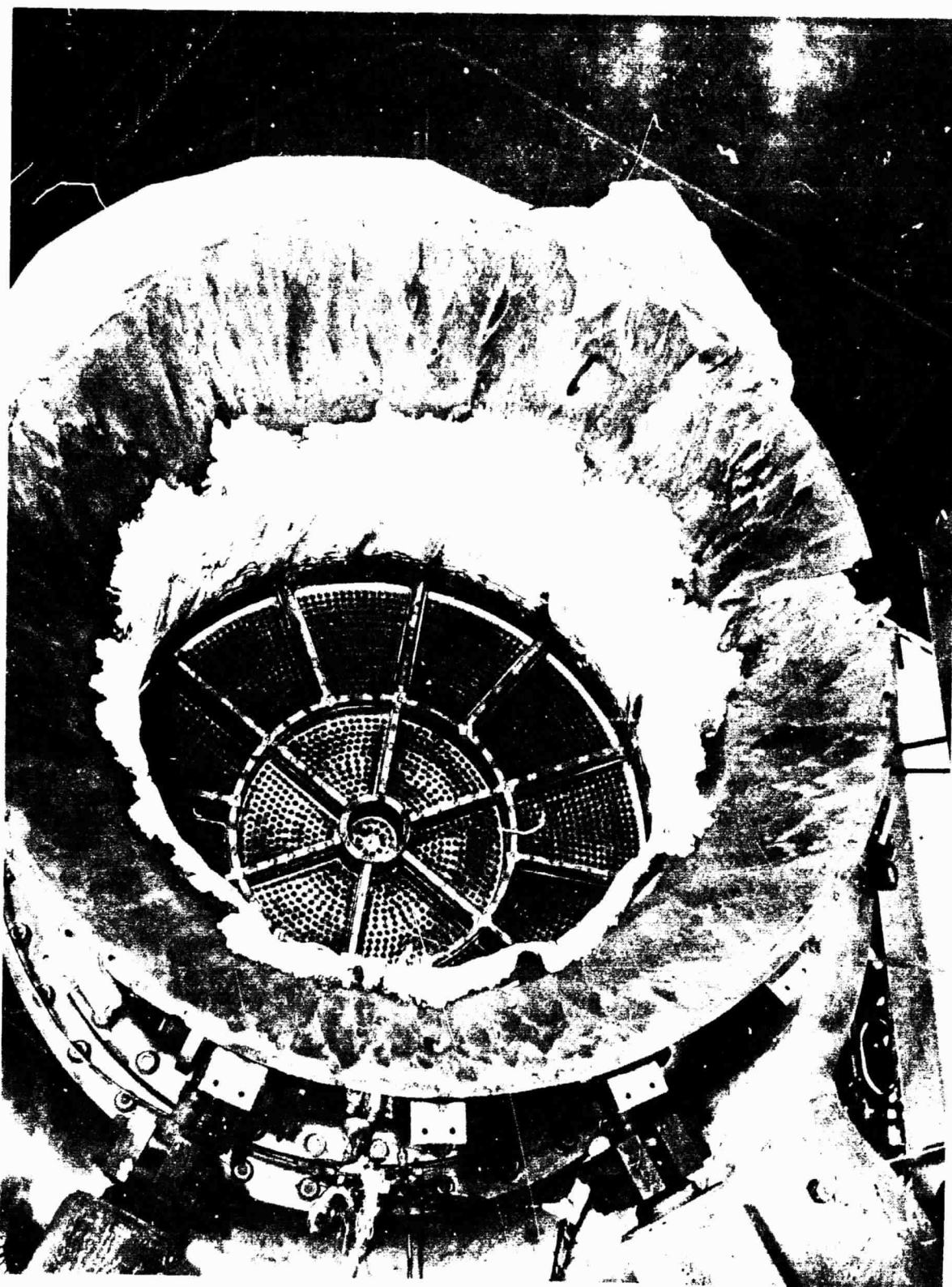
Figure 15. Damage to Nozzle Steel Shell Following Test No. 1198-D01-00-020
