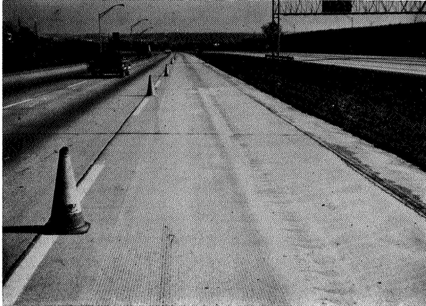
Figure 11.- Alined grooving pattern.
