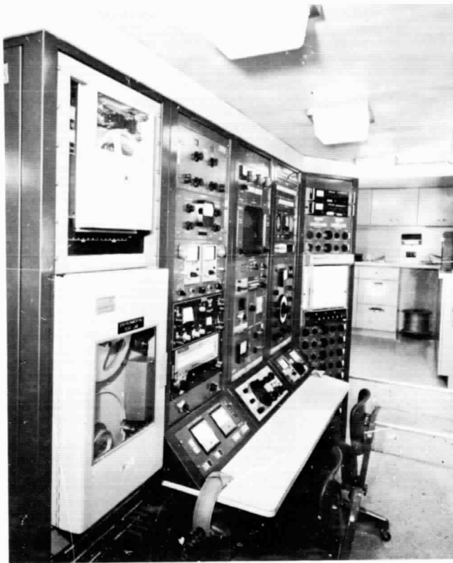
Fig. 37. Vibration control console
