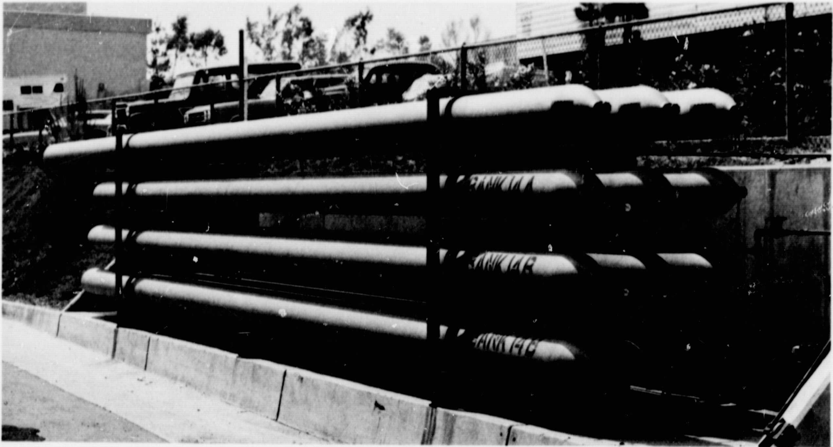
Fig. 22. Gas storage tanks
