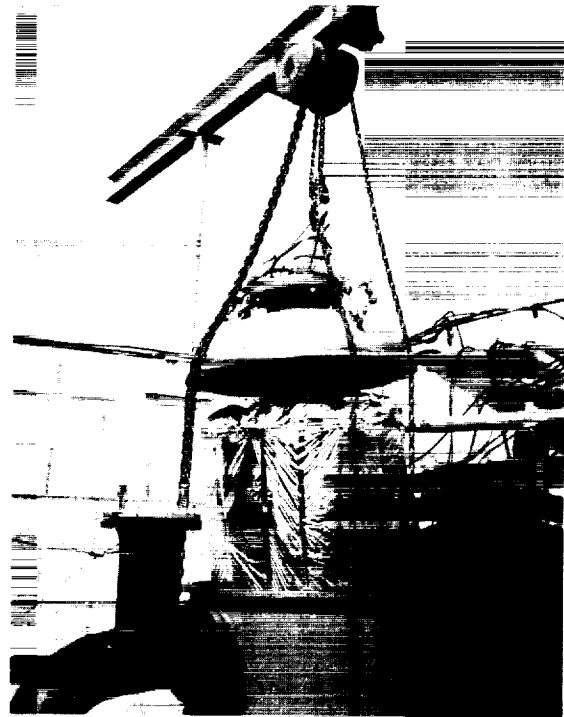
Figure 4-60. Pressure Vessel Installation in Vacuum Tank
