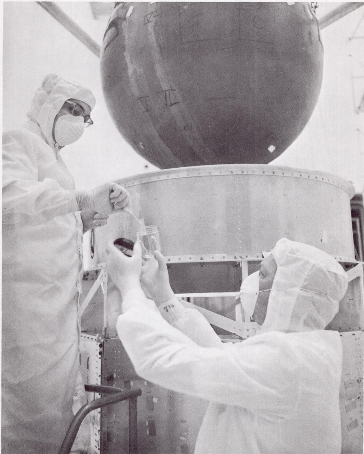
Figure 4. Sampling of Impact Limiter Prior to Being Lowered onto Payload Structure Bioengineer is Placing Coupon into Sterile Jar Held by Assembly Technician.
