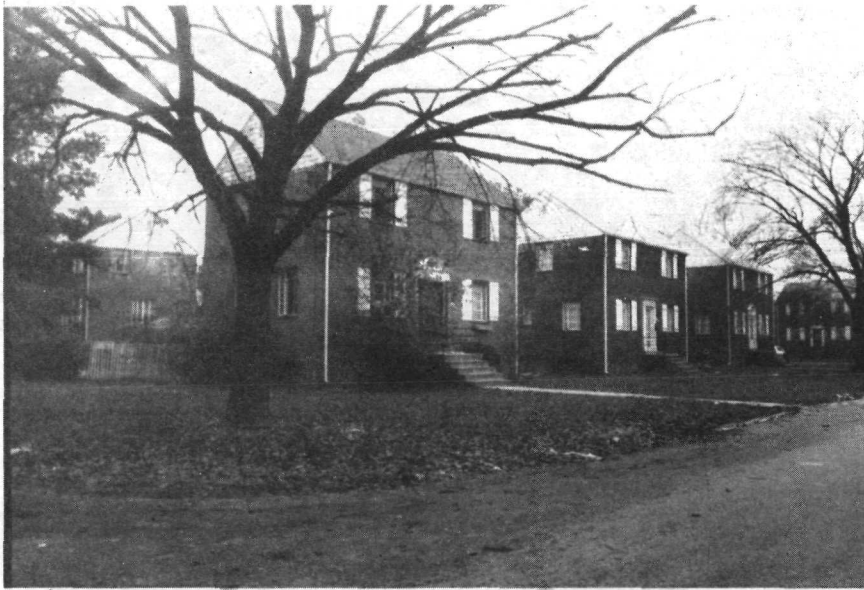
Figure 18. Census Tract #51, Detached single-family units. Masonry construction; light-colored roofs.
