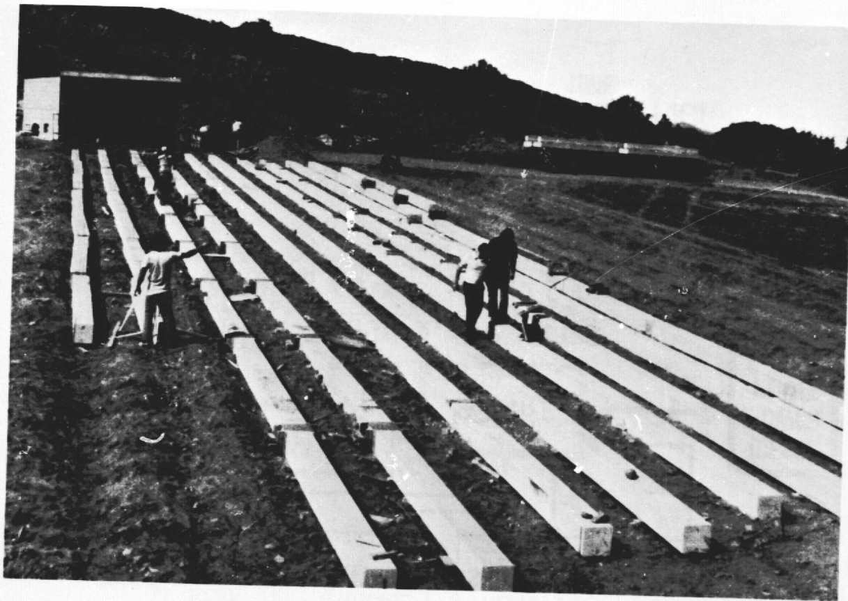
Array Foundations being Emplaced at Mount Laguna AFS
