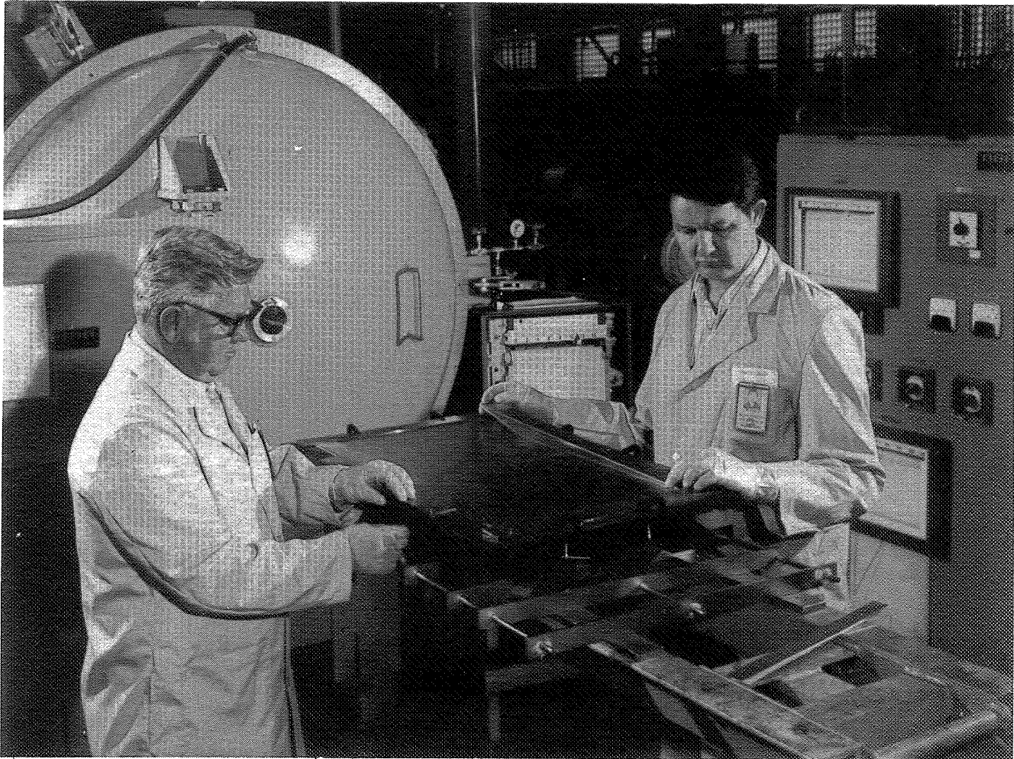
Figure 6.- Panel alinement tool.
