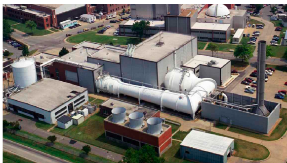
(a) Aerial view of the NTF.
