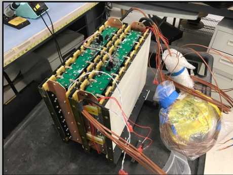
X-57 Thermal Runaway Unit (2 Trays; ½ Module)
