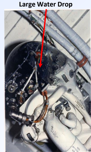
Clogged Rotary Separator on STS 32
