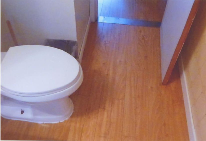
Image 1: Access to toilet on main floor
