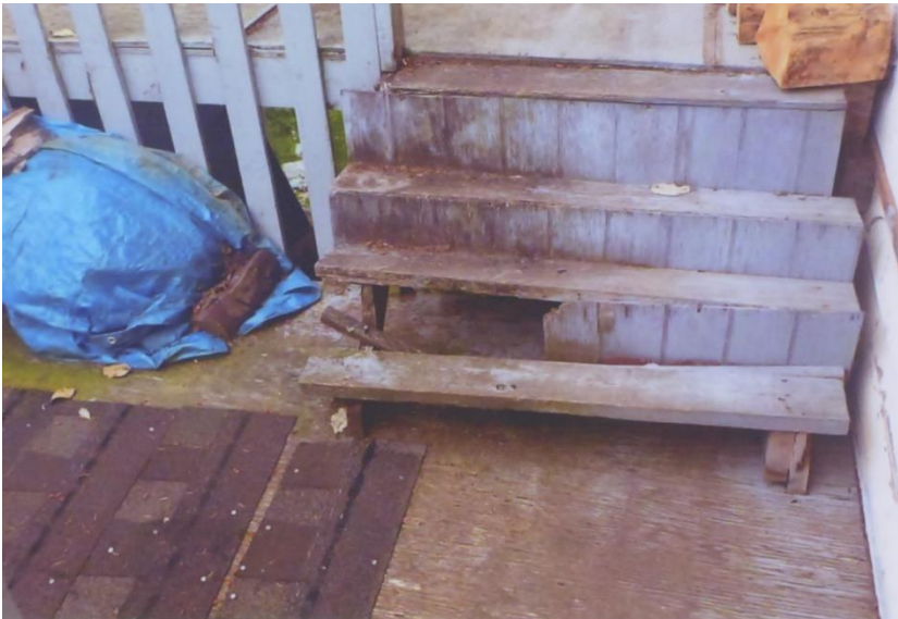
Image 4: rotten stairwell
