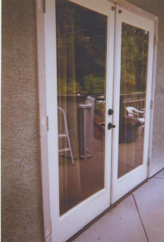
Image 3: 32” wide doorways and halls for maneuvering.
