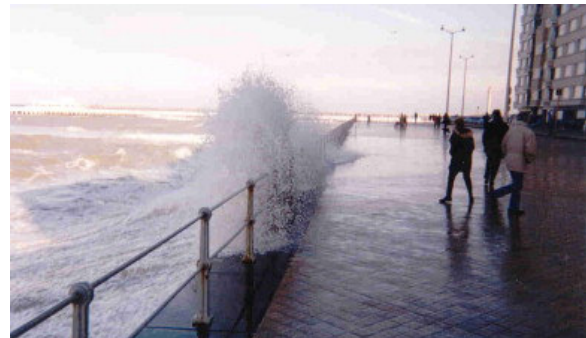
Fig. 2: Overtopping event during a storm with small return period before 2004
