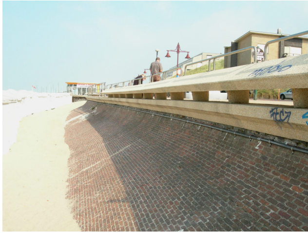
Fig. 7 - Small vertical wall at the top of the dike
