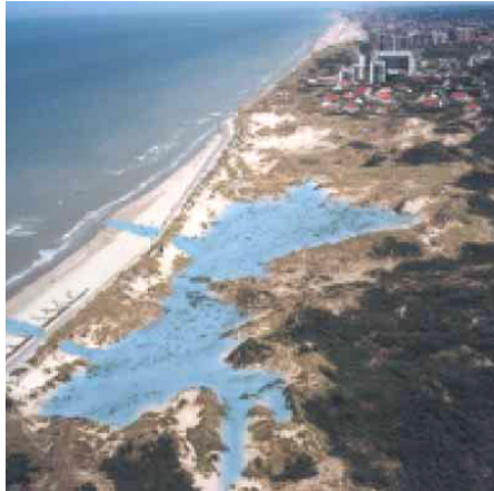
Fig. 14 - Two sea inlets (sluifers) at reserve Westhoek
