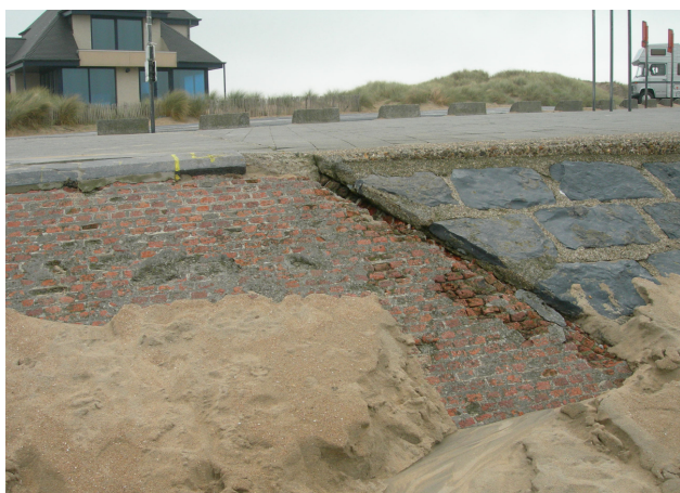
Fig. 4 - Dike made up of bricks (L), rubbles (R)
