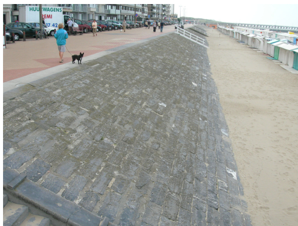
Fig. 5 - Dike made up of Tournaisian limestone
