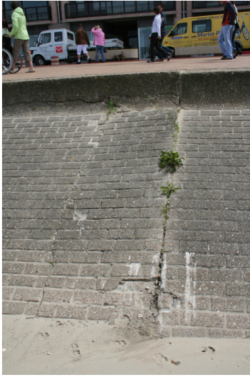
Fig. 6 - Dike made up of concrete stones
