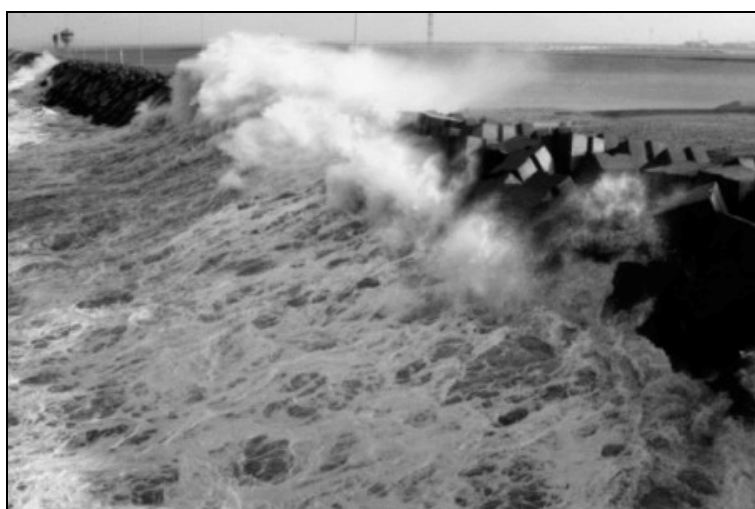
Fig. 2. Photo of wave interaction with the Zeebrugge rubble mound breakwater during storm conditions (significant wave height estimated around 3 meters).
