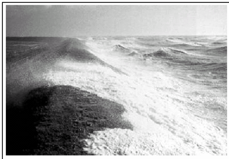
Fig. 8. A typical smooth impermeable sea dike during storm conditions.
