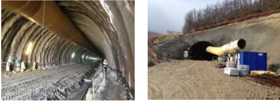
Figure 3.3: Excavation phase of the Padornelo Tunnel.
