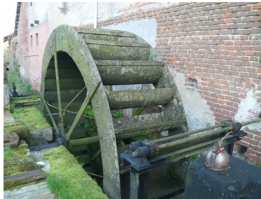
Fig. 3.1. The breastshot water wheel in Verolengo.
