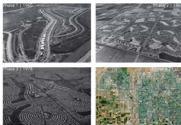
Figure 2. Sun City's the different phases of construction.
