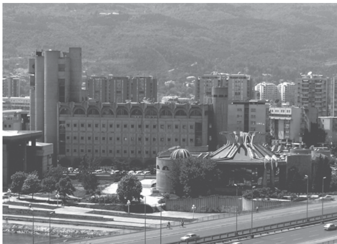
Figure 9. Panorama of the Telecommunications Centre (personal archive of Janko Konstantinov)
