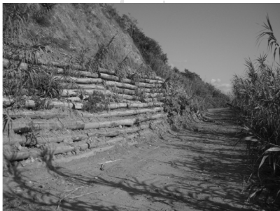
Fig. 5. (a) Filling phase and (b) placing of the upper alignments.
