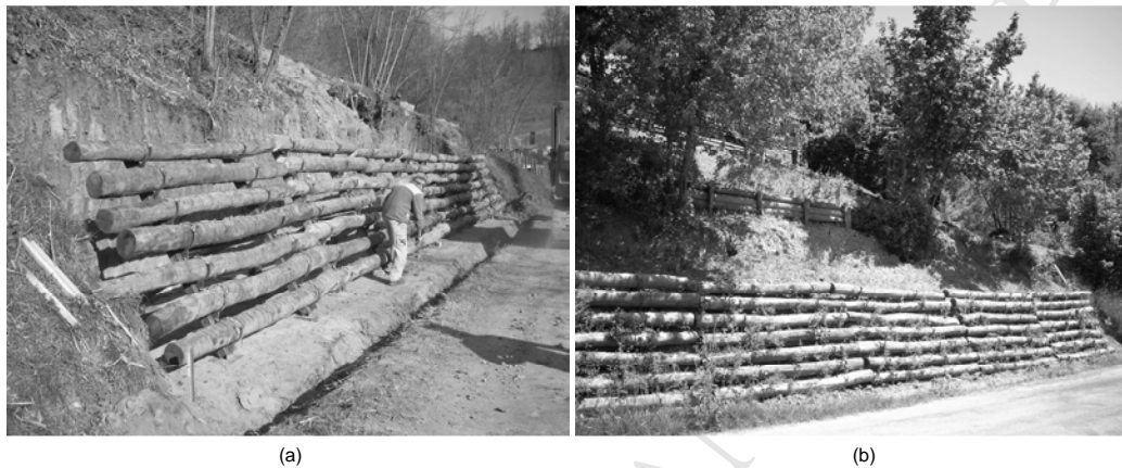
Fig. 4. Example of the structure installed at Roatto (Asti, Italy): (a) the element before the filling, and (b) final configuration when the bushes start growing.
