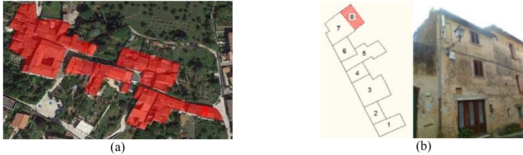
FIGURE 1. Bird-eye-view of the historical centre of San Potito Sannitico (a) and structural unit 8 of the aggregate H (b).
